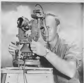
GEODESIST AT WORK: Henry A. Hook, American engineer employed by the Inter-American Geodesic Survey on a project to completely map the Americas is shown with his theodolite on top of Jamanota. On top of the instrument is the radio-controlled camera described below. TRAHADOR DI MAPA: Henry A. Hook, ingeniero Americano den servicio di Inter-American Geodesic Survey ta mantrá na trahao cu su "theodolite" na top di Jamanota.
